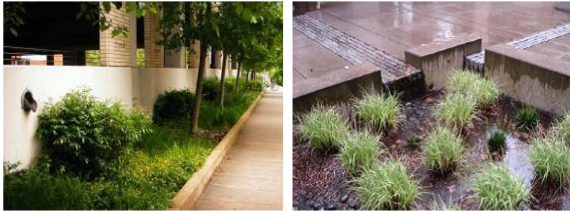
Figure 4.24-1: Various Stormwater Planters
