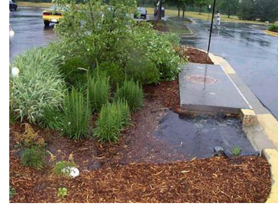
Middle Right: Figure 4.2-4 Bioretention Area after Storm
