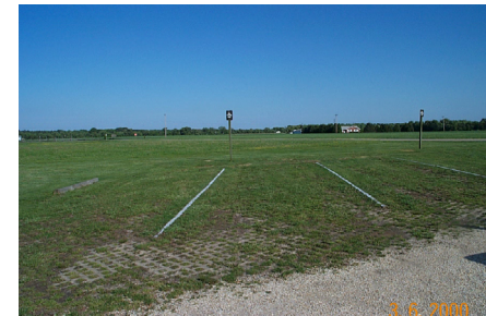
Figure 3.3-26 Permeable overflow parking area
