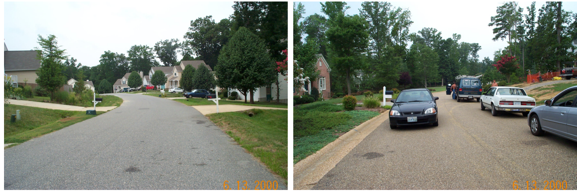
Figure 3.3-17 Narrow streets reduce impervious cover area.
