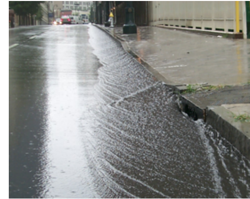
Figure 2.1-4 Impervious Cover Increases Stormwater Runoff and Pollutants
