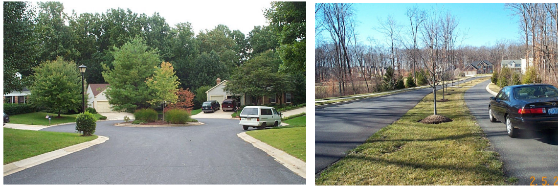
Figure 3.3-21 Cul-de-sac with vegetated island (left) and narrow road with grass swale (right).
