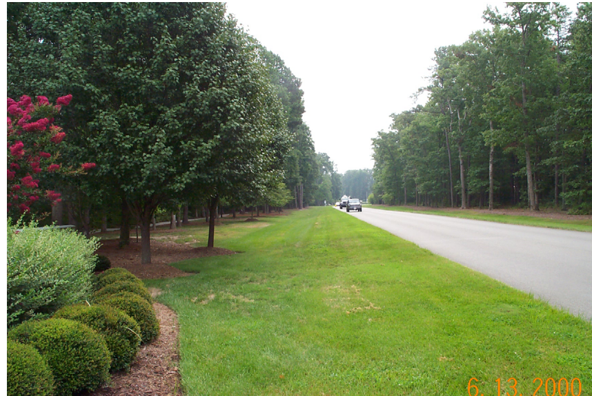
Figure 3.3-25 Road with grass swales instead of curb-and-gutter
