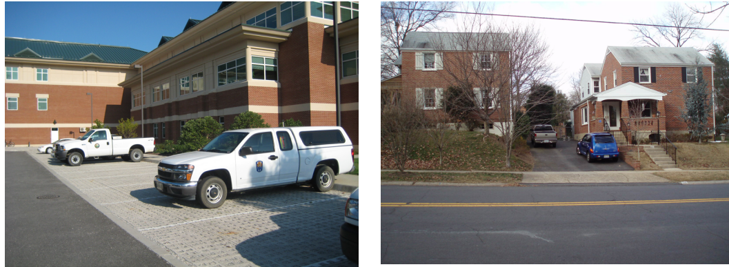
Figure 3-26 Pervious parking lot (left) and shared driveway (right).
