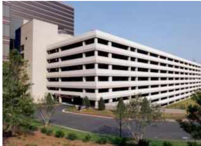
Figure 3.3-29 Building up rather than out can reduce the amount of impervious cover
