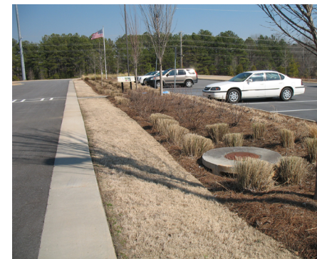
Figure 3.3-27 Parking lot bioretention in Johns Creek, GA.
