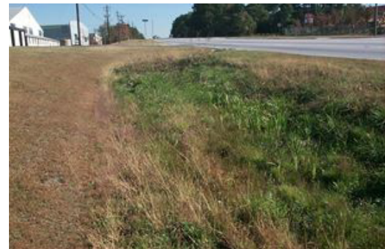
Enhanced Wet Swale
